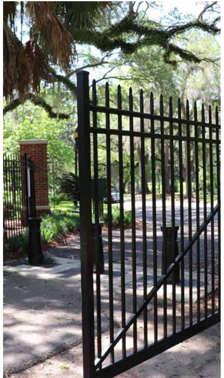
Belmont Double Swing Arch 1 Gate
